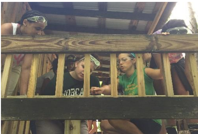
Building a bench on the front porch of a cabin
